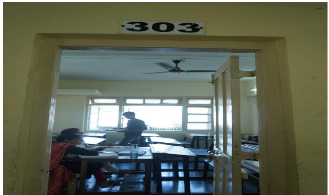
Room Room No 303 Renovation
